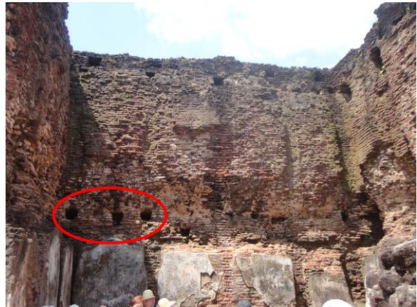
**Figure 5: Grooves which hold cross beams.**
