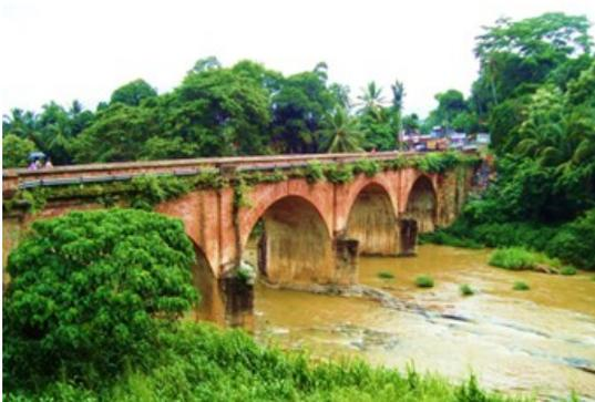
**Figure 3: Mawanella masonry arch bridge**
