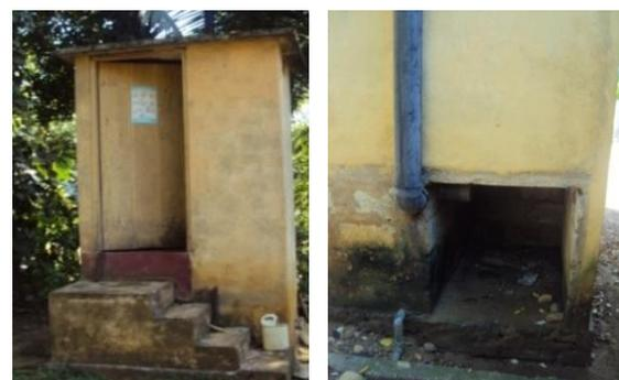
**Figure 1: eco-san toilet (left) and the collecting chamber (right)**
