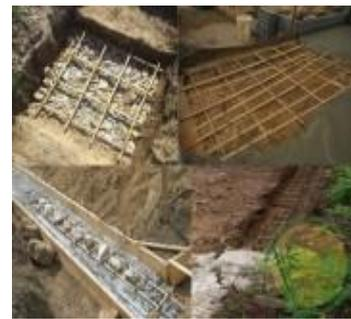
**(c). In soil-cement pavement slabs**
