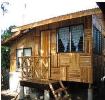
**(d). In woven reinforcing mats for wall panel construction**
