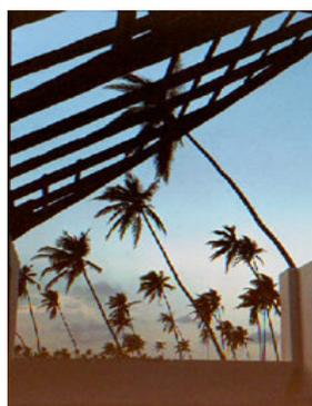
**Figure 1:** A house with a clay tiled roof. The roof covering material has completely blown away and some of the roof members have failed during the 24<sup>th</sup> November, 1978 Cyclone (Datum International)
