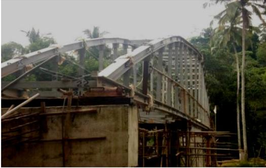
Figure 6: Ehelakanda Bridge Failure
