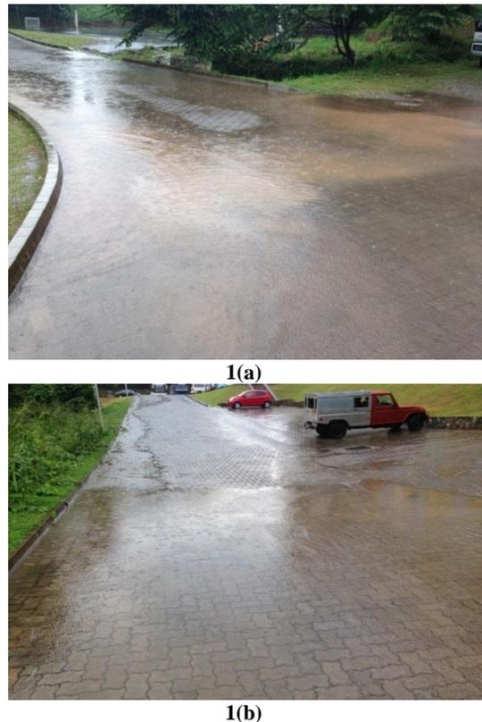
**Figure 1: Water pooling in front of Faculty of Engineering due to a small rainfall**
