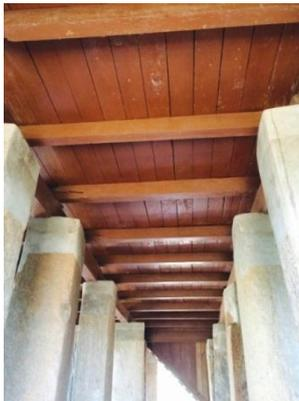
**Figure 6: Bigger columns used at the middle of the structure**
