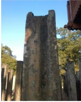
**Figure 5: Top of the columns are cut to place the wooden beams**
